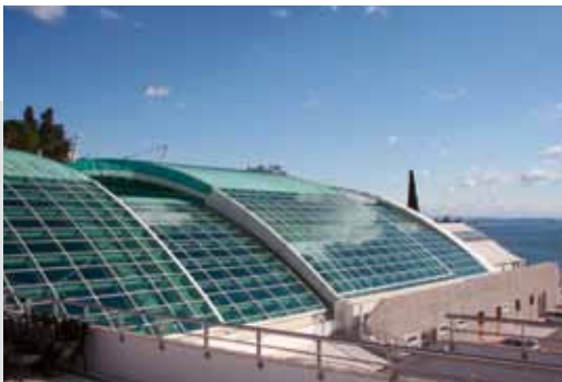
Schwimmhalle Kantrida in Rijeka, Kroatien/ Kantrida indoor pool in Rijeka, Croatia
