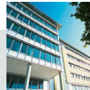
Solar-Info-Center in Freiburg
